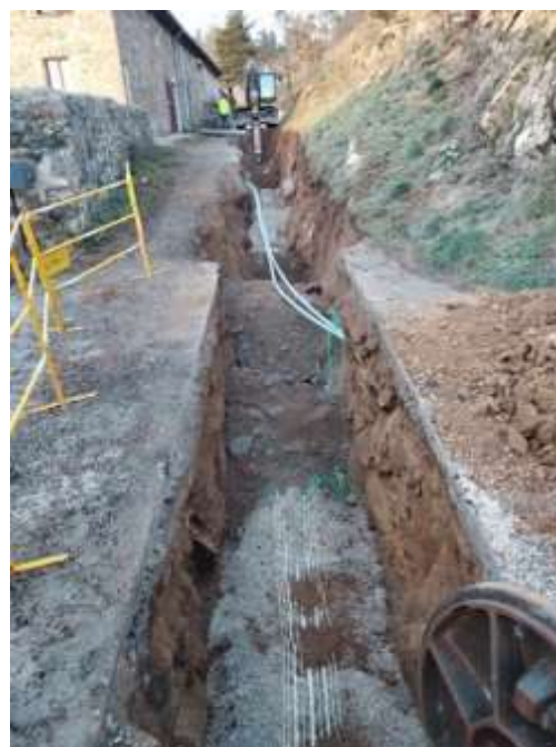
Travaux extension Champis
